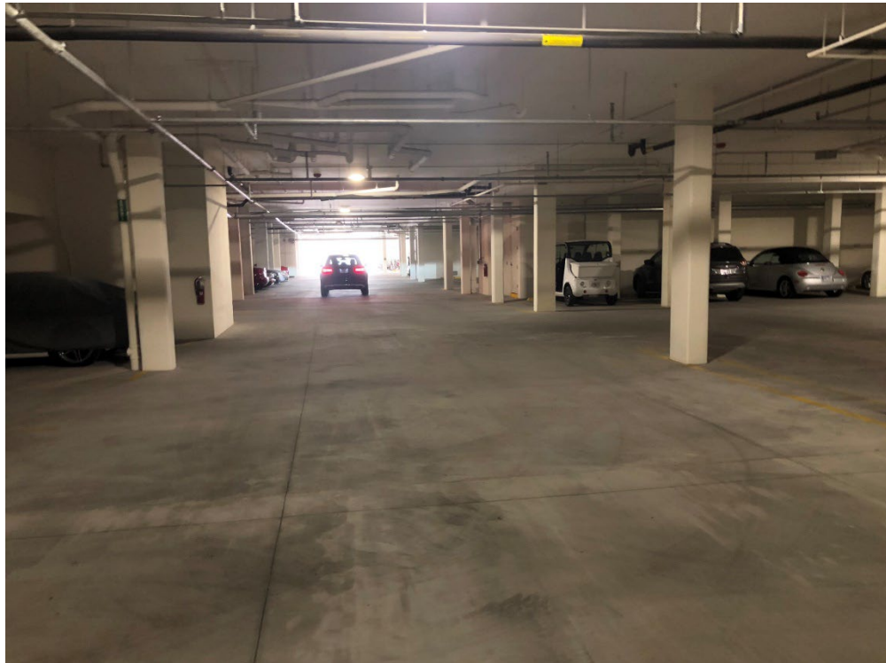
Overall view of garage interior.
