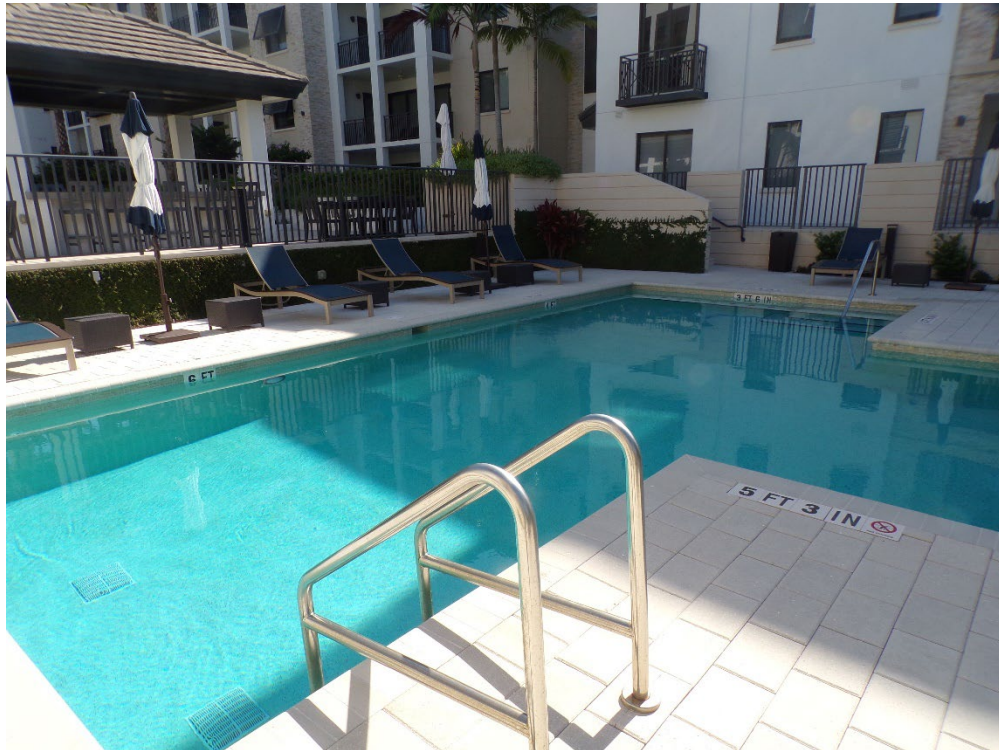
Overall view of pool deck and associated furniture.
