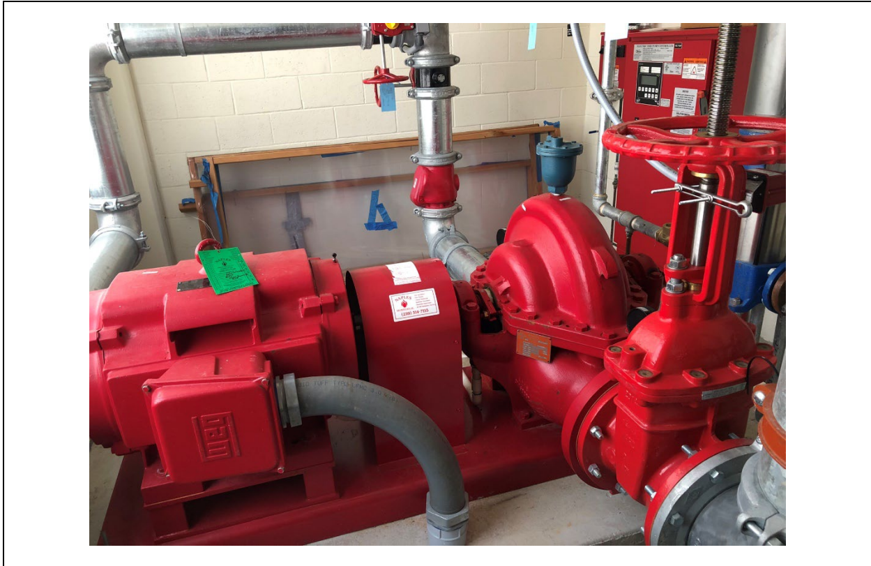
Overall view of fire pump.
