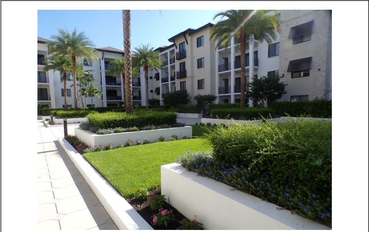
Overall view of courtyard area.
