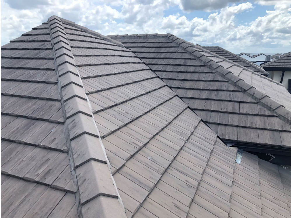
View of typical sloped, flat concrete roof tiles.
