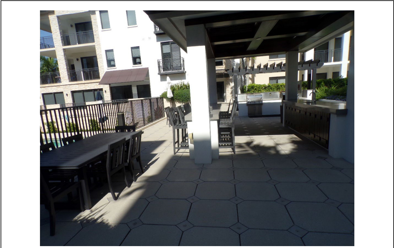
Overall view of outdoor kitchen area.
