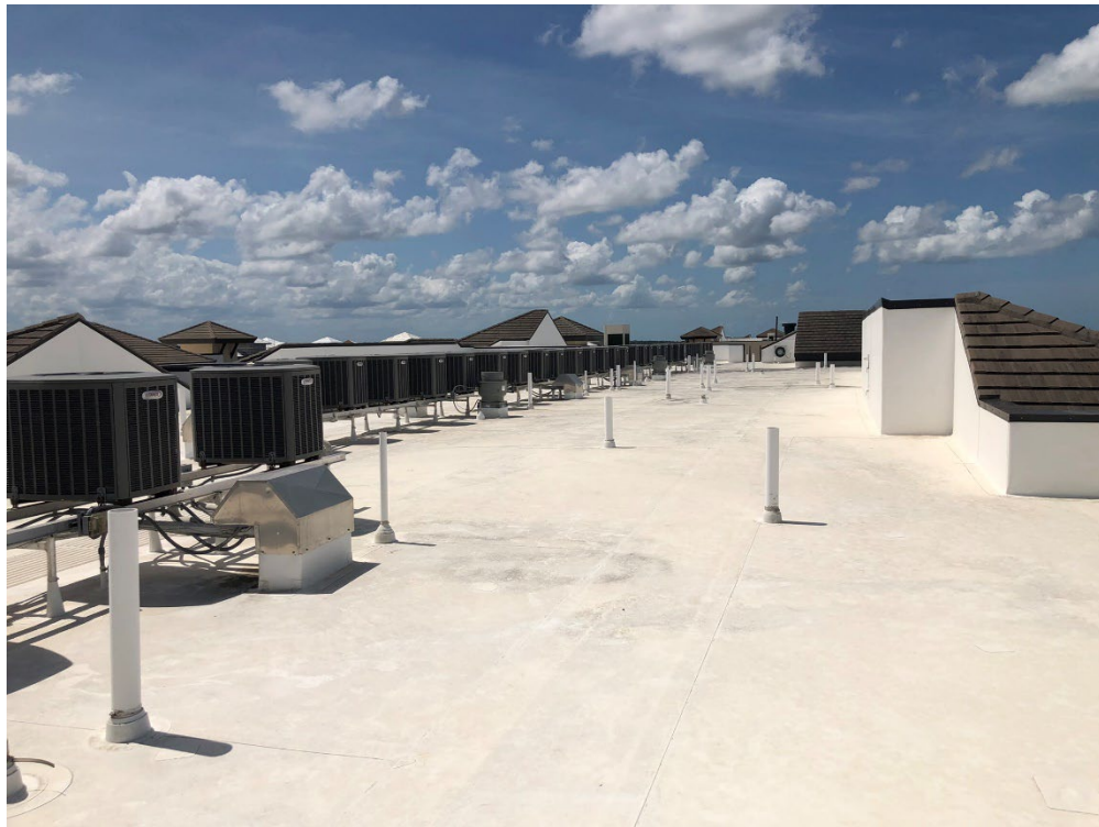
View of TPO flat roof membrane and typical metal HVAC stands.
